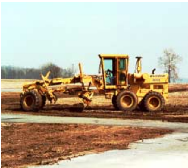
This earthmover was used to push the dirt around to level the ground around the runway and pits as well as fill a couple of low places.
